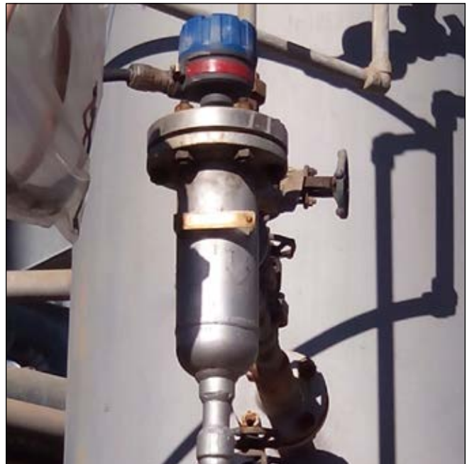
Magnetrol® Echotel® 961 mounted in an external chamber
