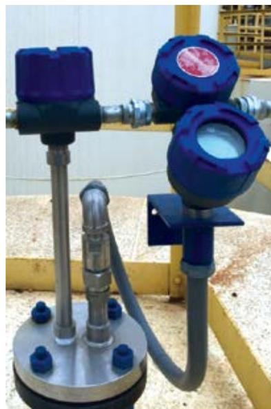
Figure 1: KMCO installation with Echotel® 961 ultrasonic high level switch (left) and Eclipse® 706 guided wave radar (right)
