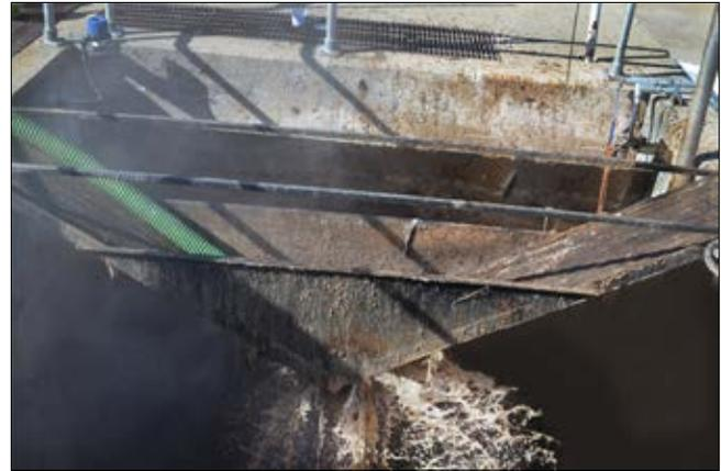
**An Echotel® ultrasonic transmitter from Magnetrol measures grease level through a fog of vapor at the WWTP grease receiving station. Grease is being fed from a tanker through the green hose.**
